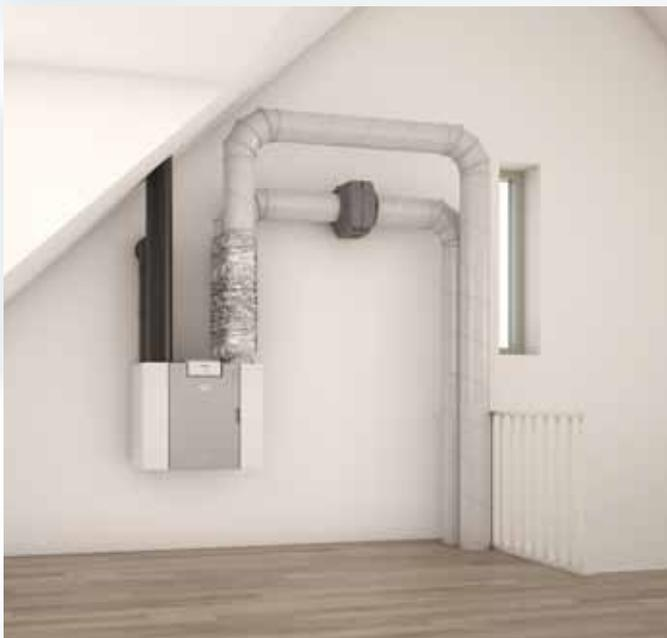
After installing the Evap in the duct from the ventilation appliance to the occupied rooms, it will be part of your ventilation system.
