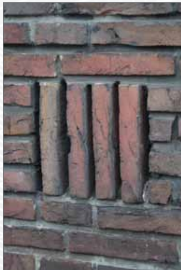
Practical example open butt joint
